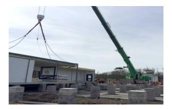
Work was completed 2017 for the extension of the existing Horizon Nuclear Power Wylfa Newydd site office; work carried out included all groundworks associated with the installation of prefabricated units to extend the overall footprint of the office.
