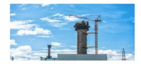
The Liebherr crane, the highest structure ever built at Sellafield, will begin work this autumn to remove and lower chunks of the chimney cut out using diamond wire saws.
