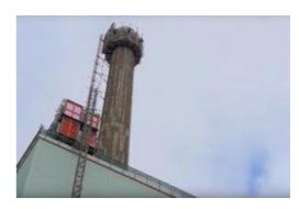
concrete crunching jaws and plasma steel cutting torches, workers will remove each piece of concrete and steel from the stack by hand to a waiting waste skip.
